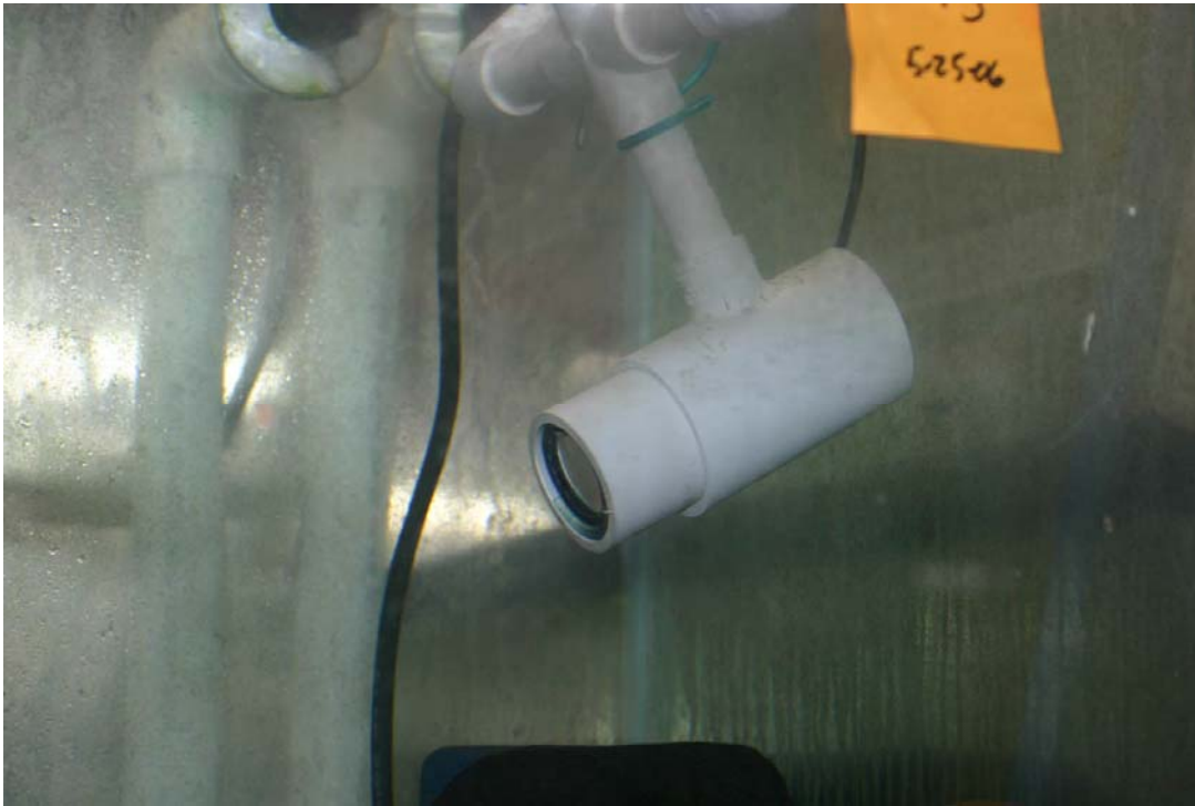
Figure 15: Micro Video MVC2000 – WP – LED digital camera being lowered into position
